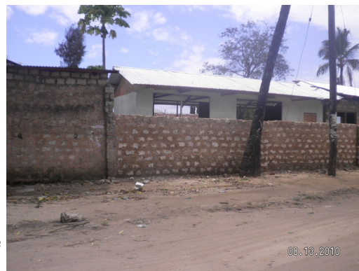
The outside wall in progress – May 2011
