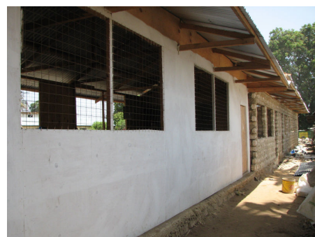
New classrooms being built.
